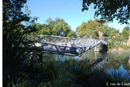
Foot bridge in downtown Christchurch
