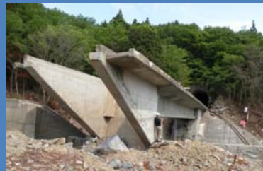
JR-Bridge at Nijyu-ichihama
