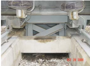
Transverse Seismic Restraint
